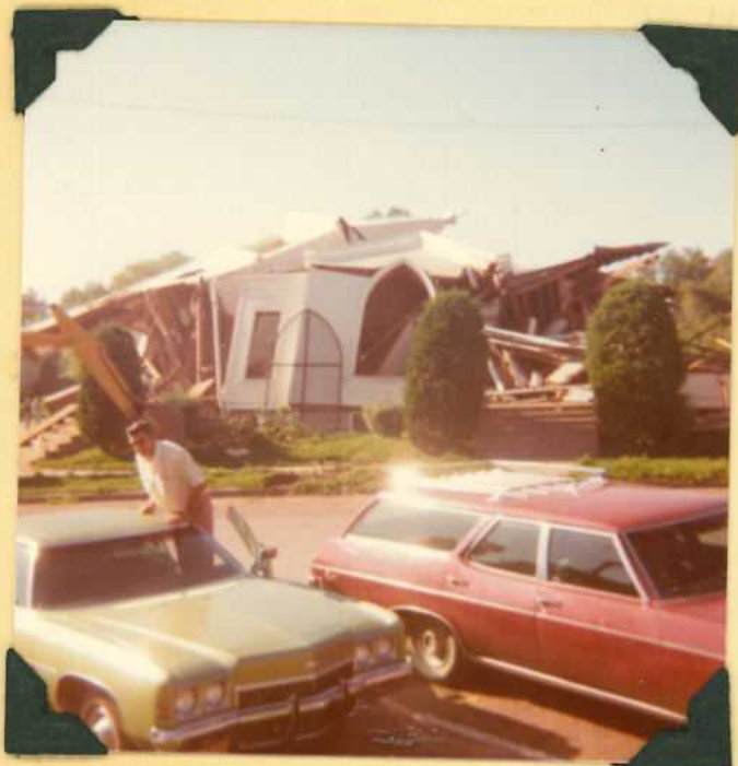
The structure shown here on its way down. It took about three jolts with the heavy boom to free this landmark from its foundation. Many sidewalk superintendents were on hand to watch Ray Hall, in the cab, give it the final blow.
